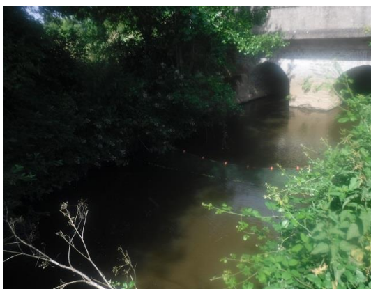
Limite amont de la station
